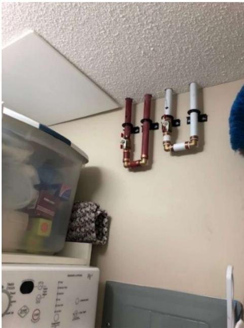
To the left is a picture and example of a water shut off valve that can be installed making it easily accessible. Many Owners have concerns that the water shut offs to their unit are either:
